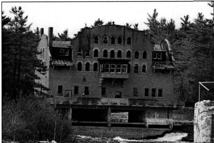
Current Image 2: McGregor Powerhouse (1922)
